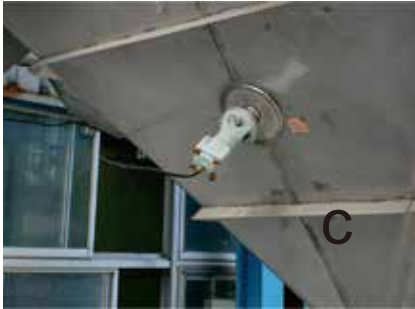
Dust collector air knocker vibrates and feeds out
