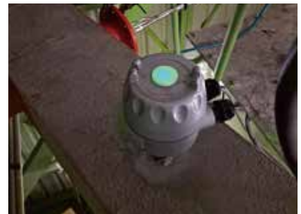
Dust collection machine dust density detection
