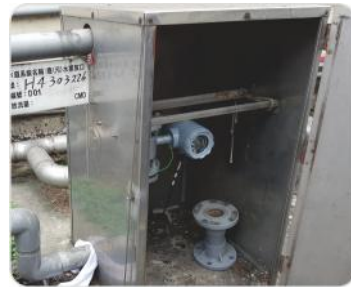
Beverage - Flow detection for wastewater discharge
