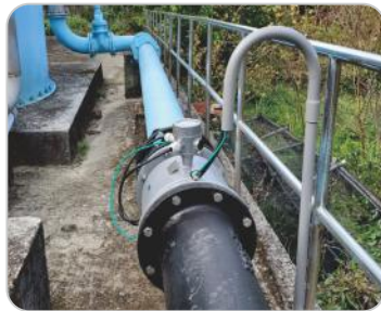
Public authority - Flow monitoring of water purification plant
