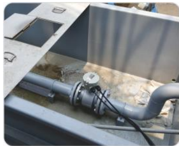
Pharmaceutical - Flow detection for wastewater discharge
