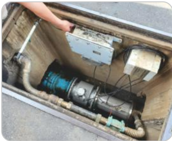
Public authority - District pipeline network of Taipei Water Department
