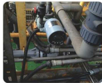
Mining - Flow detection for process water
