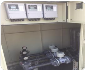
Electroplating - Wastewater discharge system
