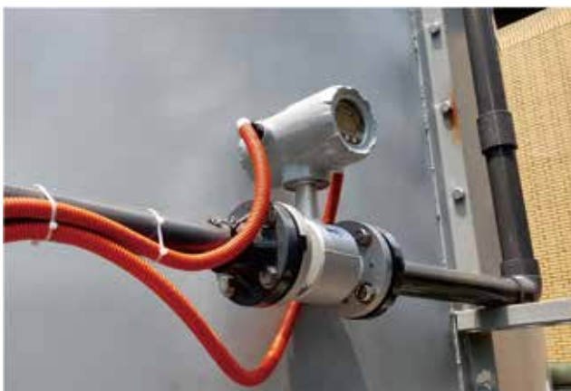
▲ Electromagnetic flowmeter
