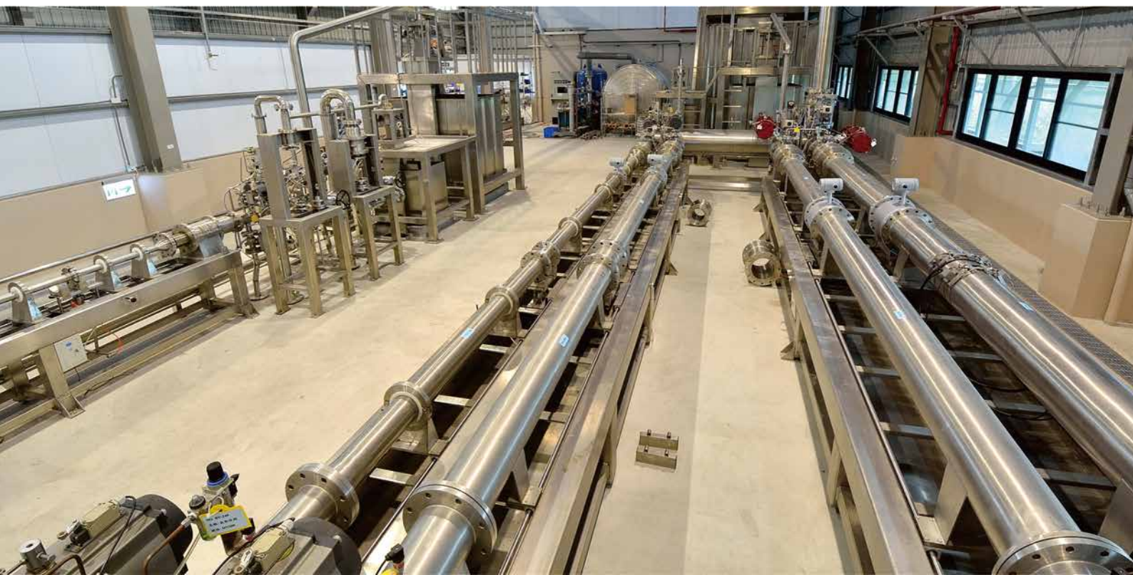
PUMP equipment (The maximum horsepower is 110KW per unit)
