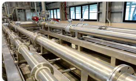
Piping system II (Maximum diameter is 500mm)
