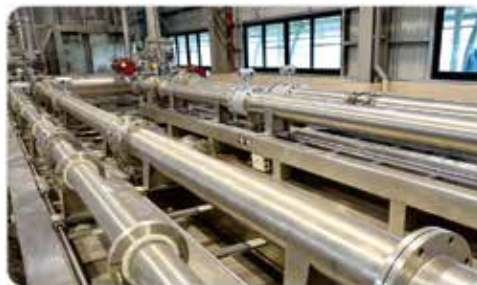
Piping system II (Maximum diameter is 500mm)
